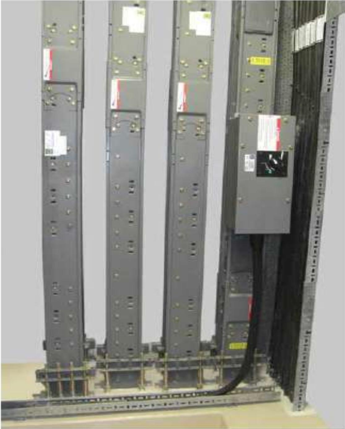
Typical busbar riser system including plug-in circuit breaker
